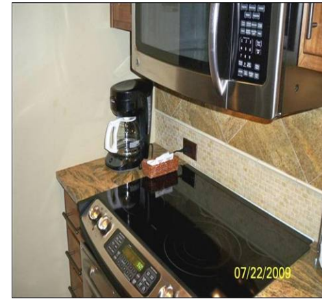
Microwave mounted beyond reach range
