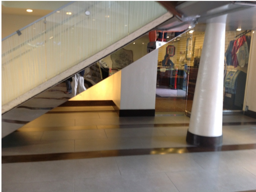
Lobby Escalator Presents A Dangerous Protruding Object
