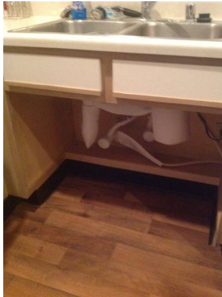
Kitchen Sink Knee Clearance and Insulation
