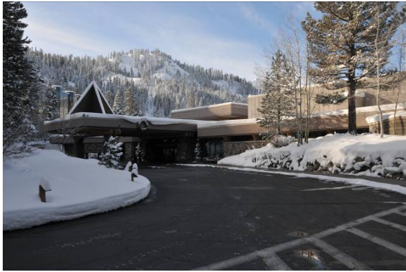
No accessible path of travel from parking spaces to entrance
